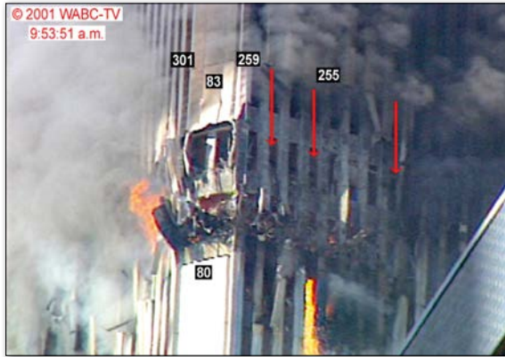
► FIG. 6: Molten metal was seen pouring out of WTC 2 continuously for the seven minutes leading up to its collapse (Sources: WABC-TV, NIST).
